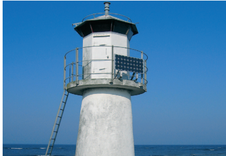
SwedModule on a lighthouse at Laus Holmar in Gotland, Sweden
